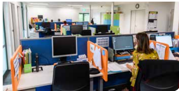
After: we've already renovated a small part of Te Whare Rānui for our community staff to work from.
